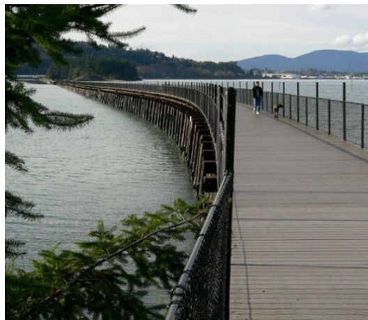
The Tommy Thompson Trail over Fidalgo Bay near Anacortes
