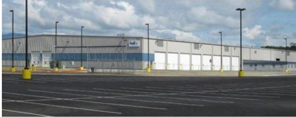
The facility acquired for Skagit Transit's Maintenance, Operations and Administration Base; Image Source: Skagit Transit Maintenance, Operations and Administration Facility Project Description
