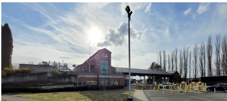
Figure 4: Kenneth G. Ward Land Port of Entry in Lynden (Source: General Services Administration)
