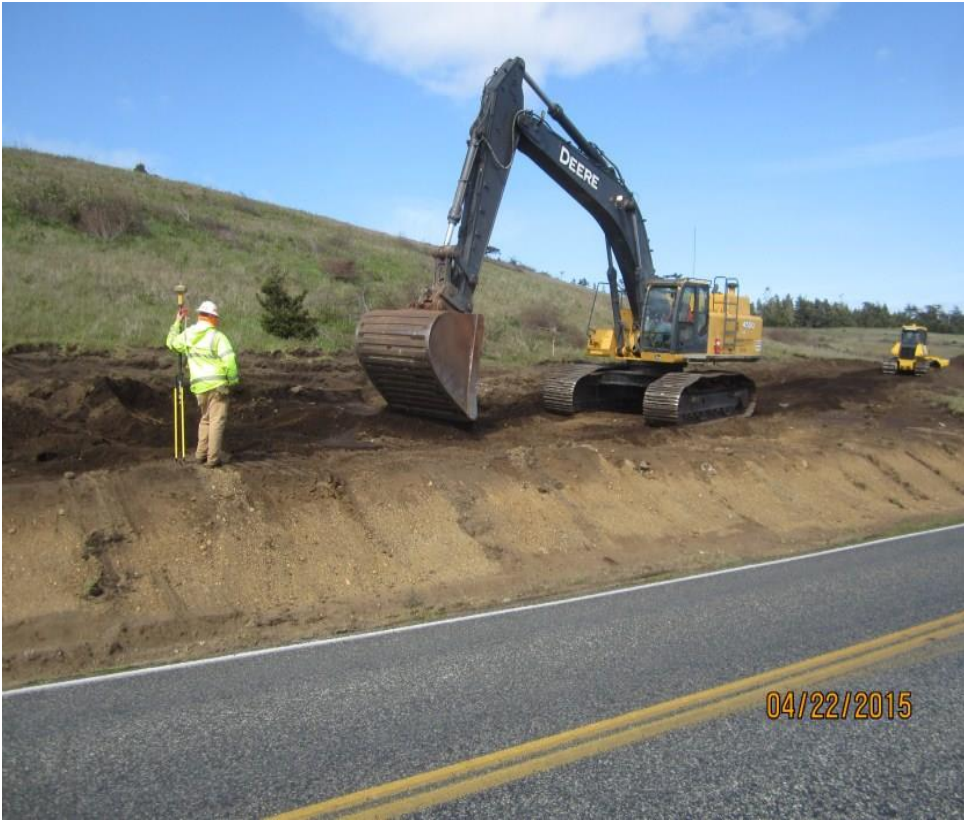
Ongoing construction at Cattle Point Road. (Courtesy FHWA)
